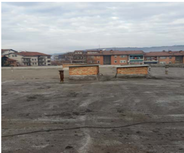
Brick and galvanized vents
