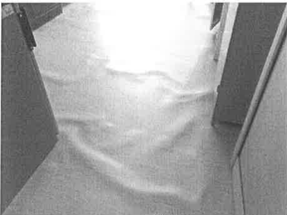
Deformations on PVC floor in the Agro-Chemical School
